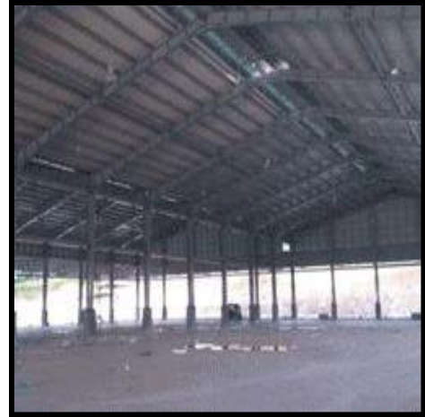
UNDER BUILD ERECT CORPORATION Bacolod Tanduy Boiler Warehouse Murcia, Negros Occidental
