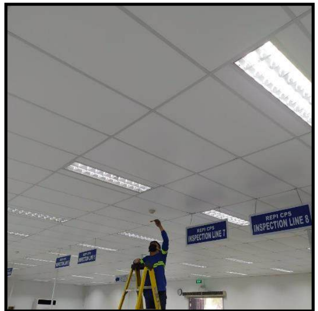
FDAS INSTALLATION PTC Nep Logistics Inc.
