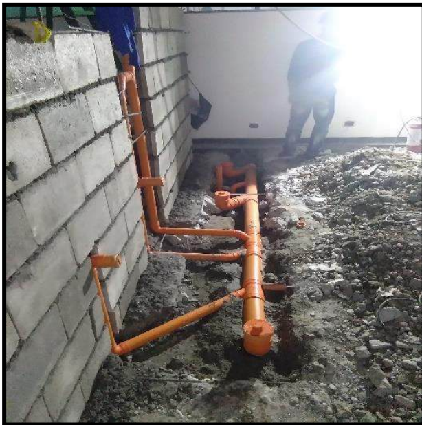
SEWER & DRAINAGE LINE IMI Laguna Technopark Phase 5 Binan, Laguna.
