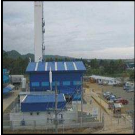
AIR SEPARATION UNIT PLANT (ASU) Southern Industrial Gases, Inc. (now Linde Southern Phils., Inc.) CIPDI, Buanoy, Balamban, Cebu
